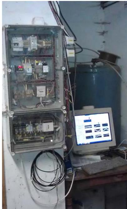
Figure 5: Control cabinet, and PC running National Instruments LabVIEW software for monitoring and control.
